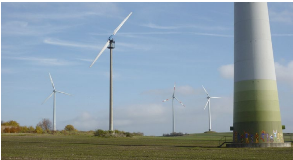
The Dardesheim wind farm has grown organically over the past two decades, and turbines continue to be gradually added. Visiting the wind farm is like going to a wind turbine museum. At the bottom of the tower on the right, local children were allowed to paint life-size figures. Photo: Craig Morris
