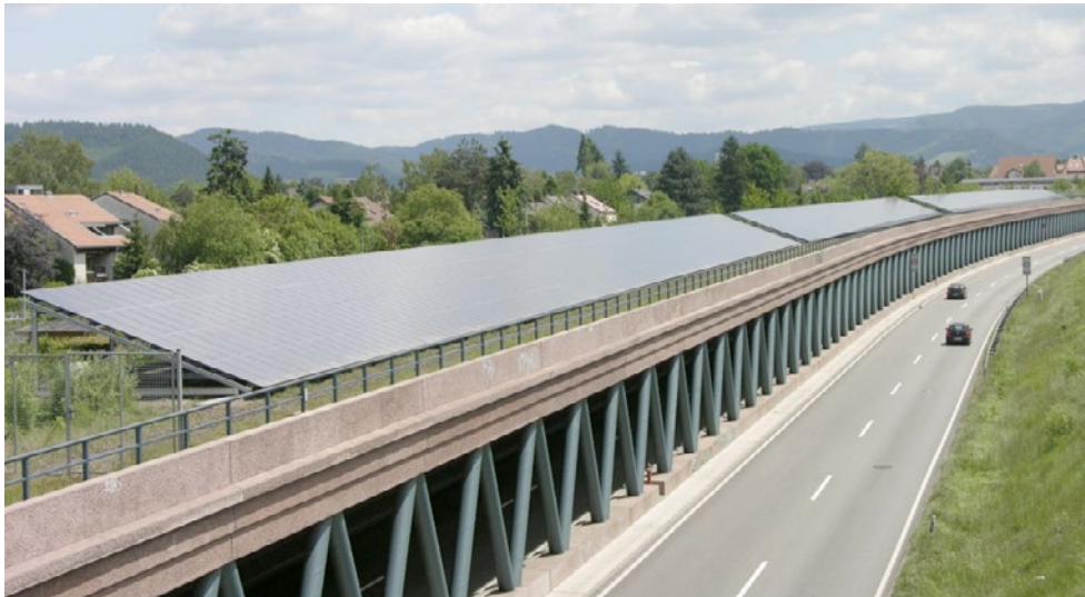
A community-owned PV array on a noise barrier in Freiburg, Germany. Source: fesa GmbH 2006
