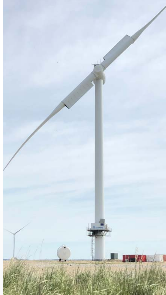
Envision's GC1-Turbine in Thyborøn, Denmark. The superconducting generator was mounted and tested on this turbine. Photo: THEVA
