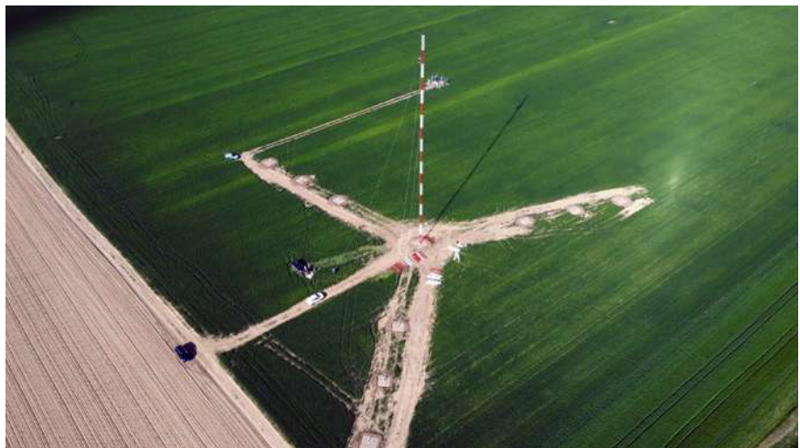
Installation of wind met mast
