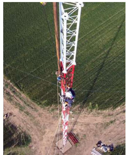
Installation of wind met mast
