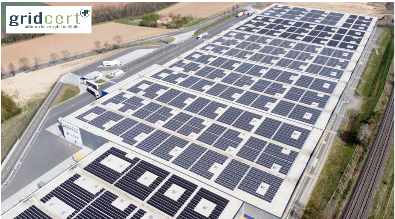
Photovoltaic project in Monsheim – implemented with the “gridcert” AI platform. Photo: Wirsol
