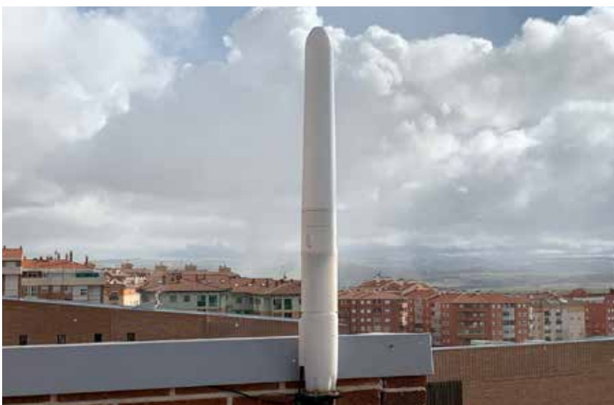
A Vortex Bladeless plant is producing electricity on the roof of Ávila University. Photo: Vortex Bladeless
