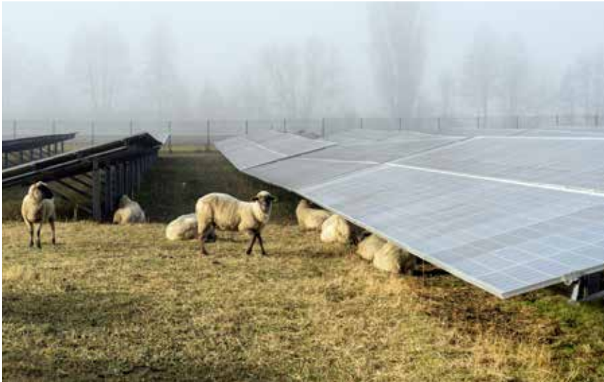
Solar Park Vogtsburg Citizens' Energy Cooperative. The energy cooperative owns 75 percent of this solar park with 7.7 MW peak power and 31,000 solar modules. The remaining 25 percent are owned by FS Solar Concept. Photo by Paul Langrock.
