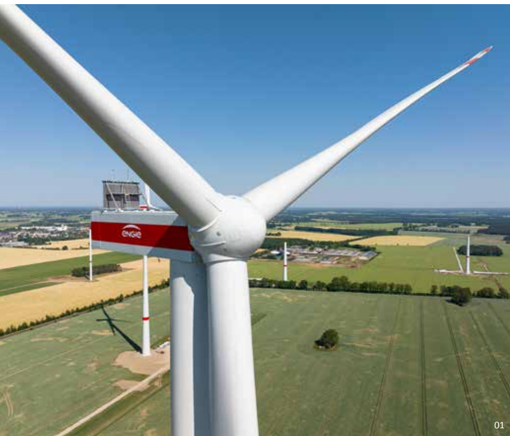
01 | Repowering Karstädt wind farm (Brandenburg) 02 | Dismantling of old plants, Karstädt
