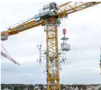
Wind turbines on the construction crane of SÜBA AG in Stockerau
