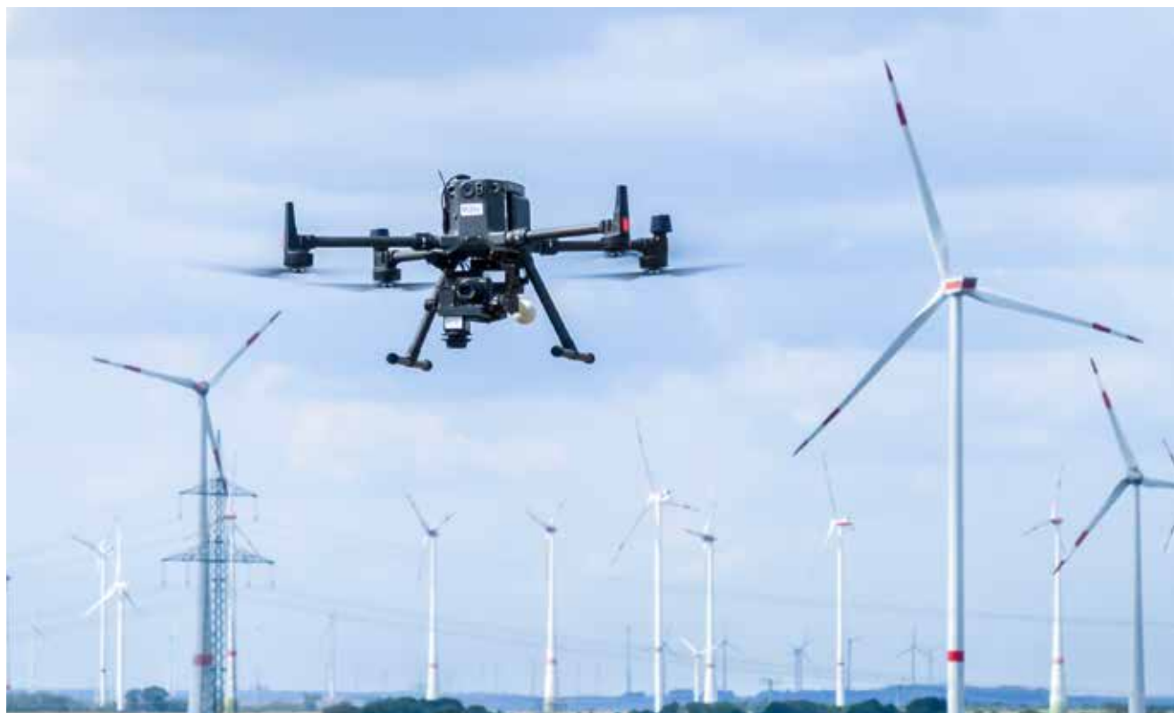
Initialization successful: visual drone inspection creates images in high definition quality, allowing for identification of damaged areas in the 1–2 mm range. © ENERTRAG / Silke Reents
