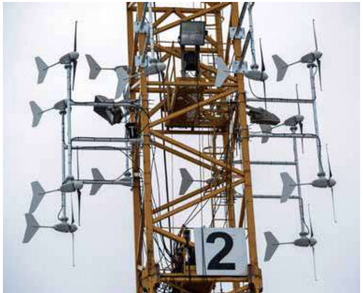
Close-up view of wind turbines on the construction crane of SÚBA AG in Stockerau
