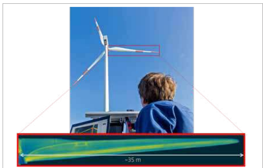
Fig. 1: Visual depiction of the internal structure, based on thermal inspection of rotating wind turbine blades. Source: BAM
