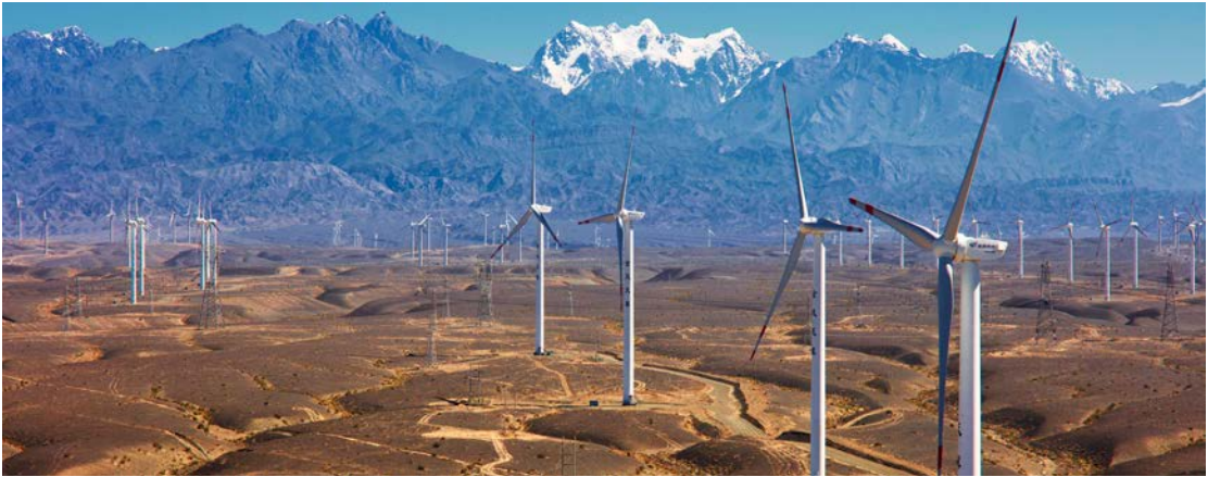
Project in Dabancheng, Xinjiang, China. Photo: Goldwind
