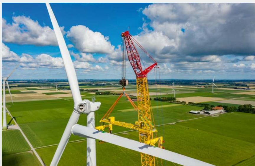
New HP generator, new nacelle design (faster assembly; more common parts). Photo: Klaas Eissens
