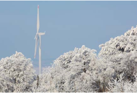
Ice on the rotor of an Enercon E-40 at Breitenau wind farm. Photo: Jan Oelker
