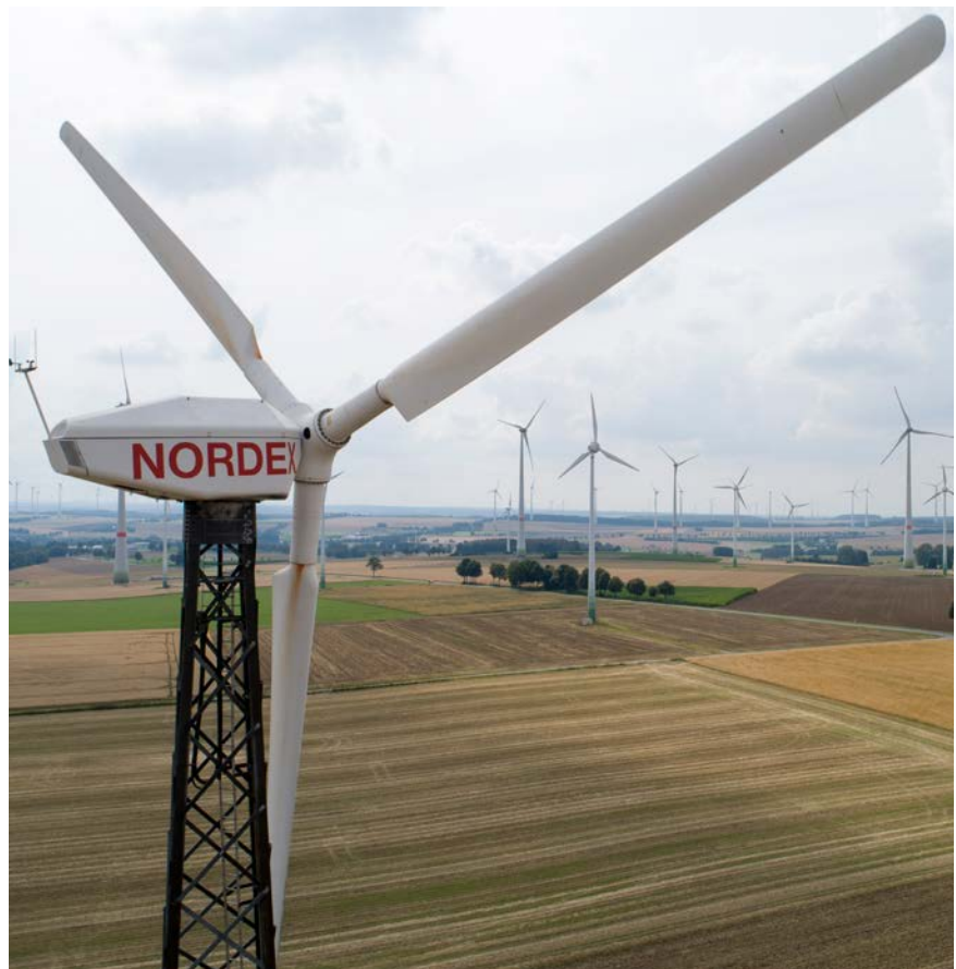
Nordex lattice tower wind turbine at Lichtenau wind farm in Asseln. Photo: Ulrich Mertens
