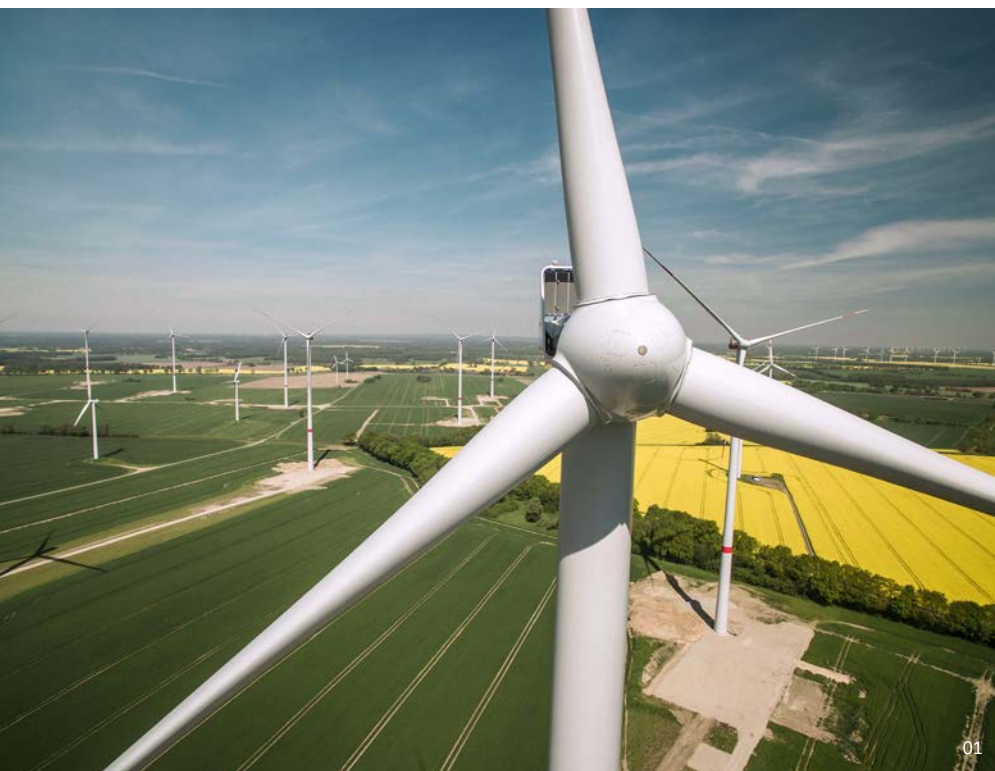
01 | Wind farm repowering project Vormark/Prignitz, Brandenburg: After dismantling the old turbines 14 new turbines were erected (nominal output of 48.3 MW).
