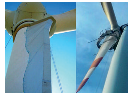
Installing the EvoFlap
