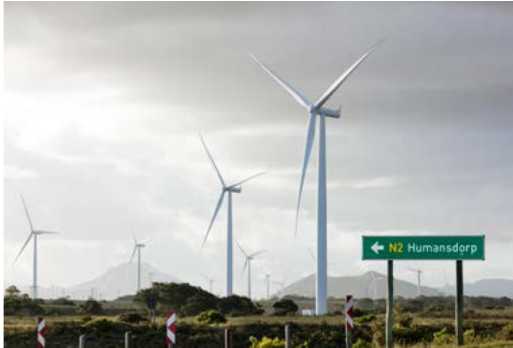
Jeffreys Bay wind farm, South Africa, with 60 SiemensGamesa wind turbines. Photo: Paul-Langrock.de
