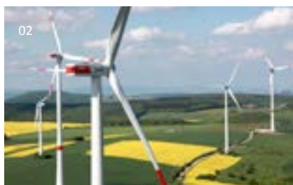
01 | Competent, experienced and passionate: project development of juwi Group 02 | Windpark Lettweiler Höhe (Rhineland-Palatinate): Repowering-Project with public participation on heights in Southwest.
