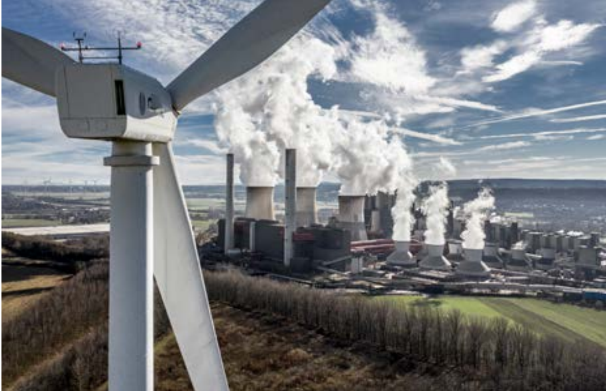
RWE lignite power station in Weisweiler. Photo: Paul-Langrock.de
