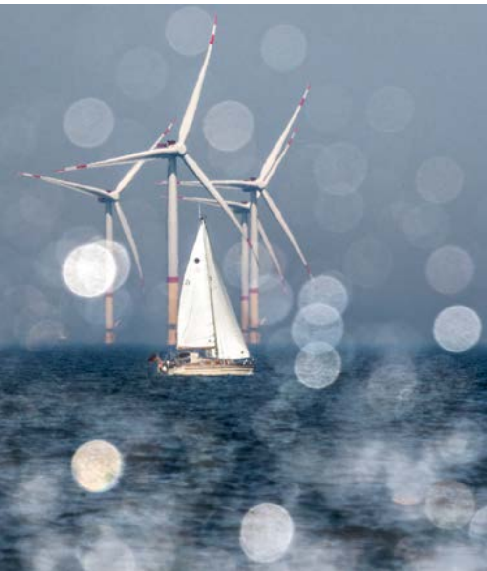
The 60 turbines of E.On's Arkona offshore wind farm in the German Baltic generate a total output of 384 MW. Photo: Paul-Langrock.de
