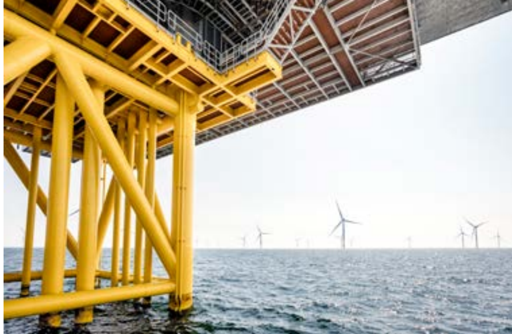
View from the transformer station at Arkona offshore wind farm. Photo: Paul-Langrock.de
