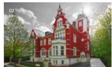
02 | Headquarters of NOTUS energy in Potsdam
