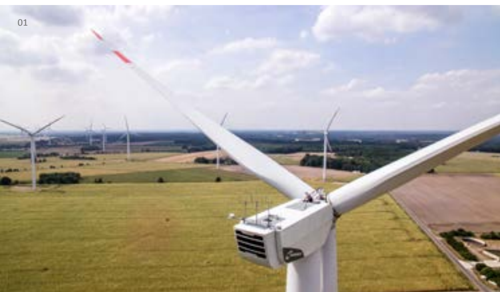
01 | Wind farm Hamwiede (Germany) 02 | Rotor blade heavy load Dachsbach (Germany) 03 | Heavy load with own truck fleet 04 | Wind farm Oberwohld (Germany)
