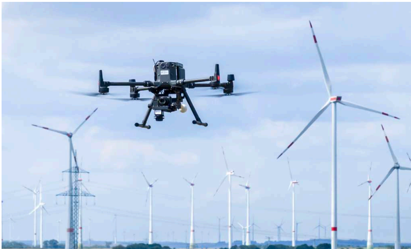
Initialization successful: visual drone inspection creates images in high definition quality, allowing for identification of damaged areas in the 1–2 mm range. © ENERTRAG / Silke Reents
