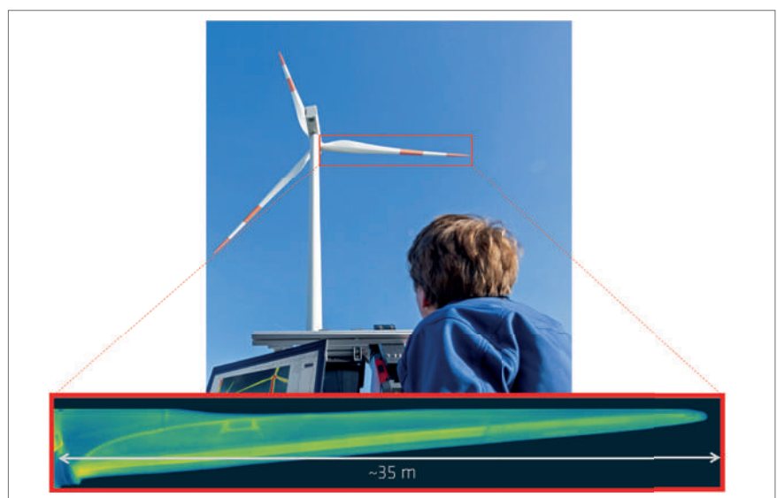
Fig. 1: Visual depiction of the internal structure, based on thermal inspection of rotating wind turbine blades. Source: BAM
