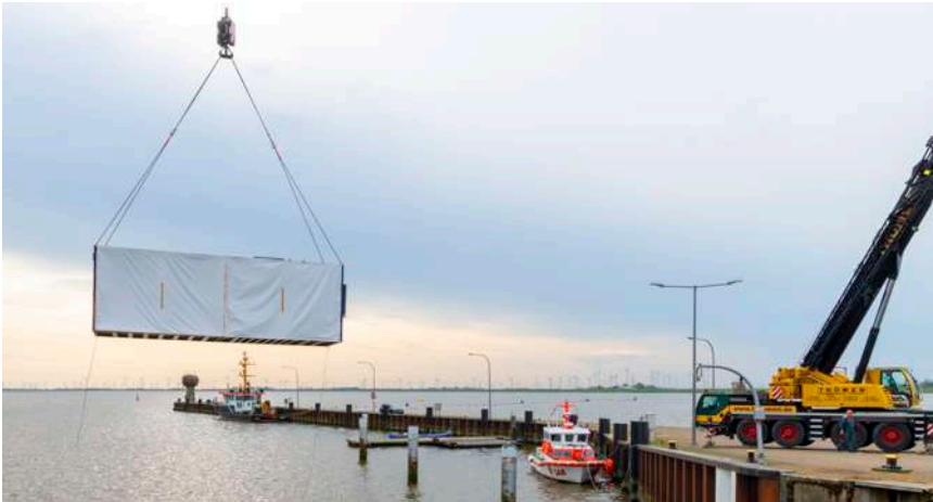
Moving the corrosion protection metrology container from BAM TTS to the Eider barrage location Source: BAM
